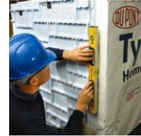
Pre-molded panels are installed level and secured with stainless steel screws.
