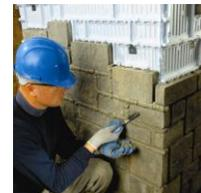
Mortar is applied using manual gun. Joints are finished & excess mortar is removed.
