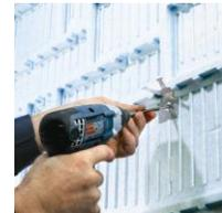
Anchors hold polystyrene panels in place and secure masonry to frame of house.
