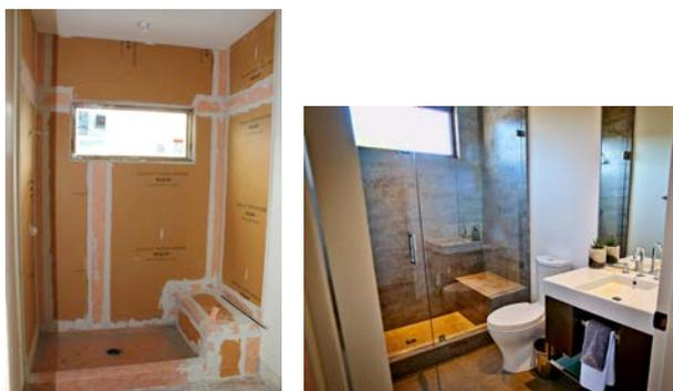
**Schluter®-KERDI-BOARD** was used on the shower walls in VISION House Los Angeles as shown in these before and after photos in one of the bathooms. [Photo on far left courtesy Structure Home. Photo on left by lathamarchitectural.com]
