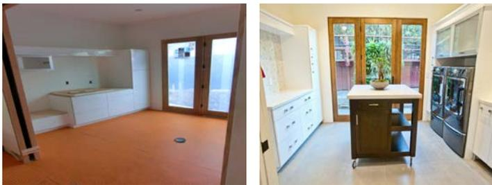
**Schluter®-DITRA** [far left - photo courtesy Structure Home] is shown in the installation phase in the laundry/mudroom of VISION House Los Angeles. The finished product is shown [left - photo by lathamarchitectural.com] with ceramic tile installed over the product.
