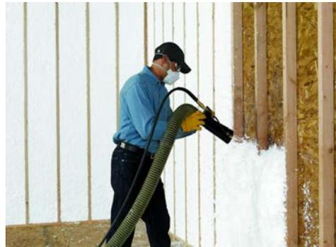
Johns Manville Corbond MCS SPF closed-cell spray polyurethane foam in the roof brings its R-value to 38 (at 6" thickness). Johns Mansville blown-in Spider insulation makes for an R-19 wall.
